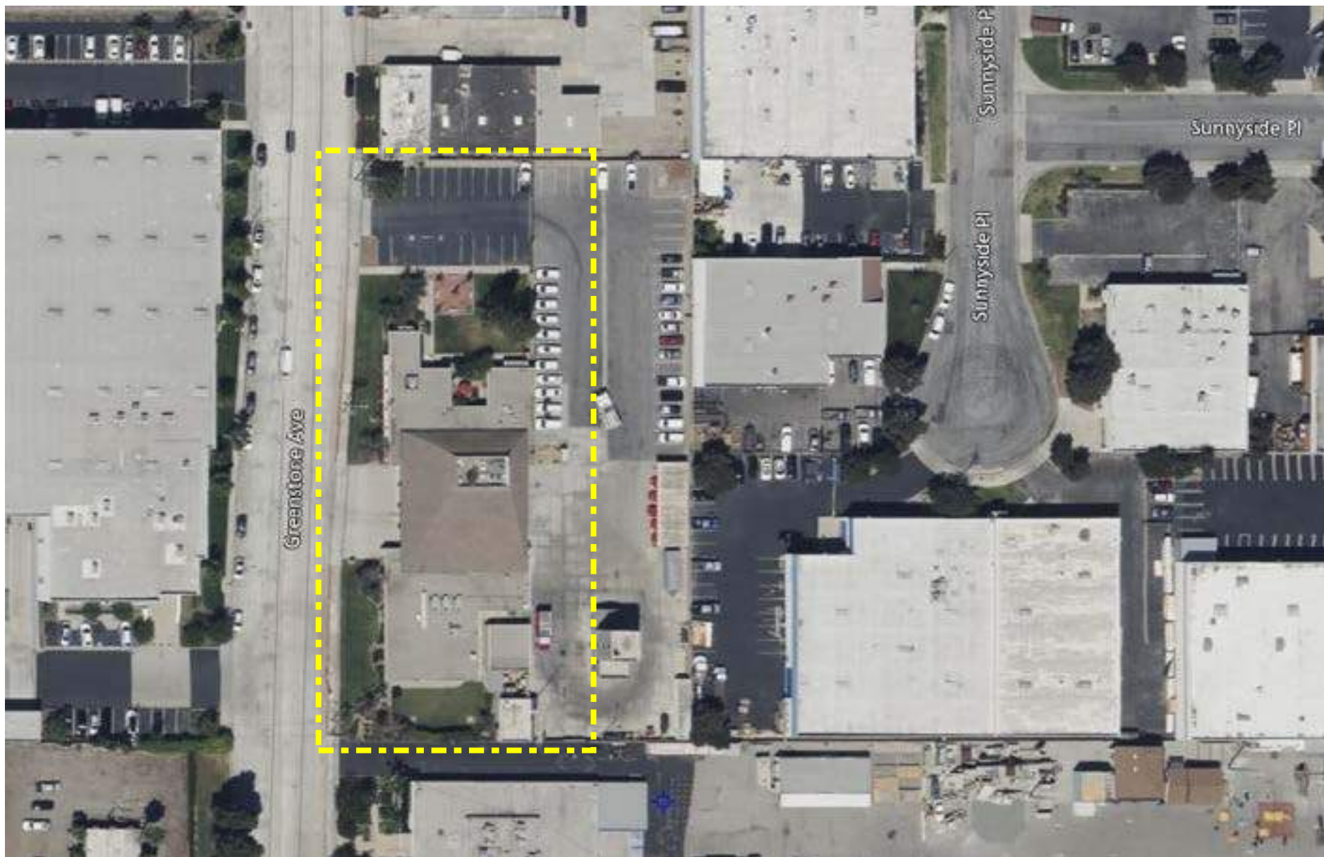
FIRE STATION HEADQUARTERS
