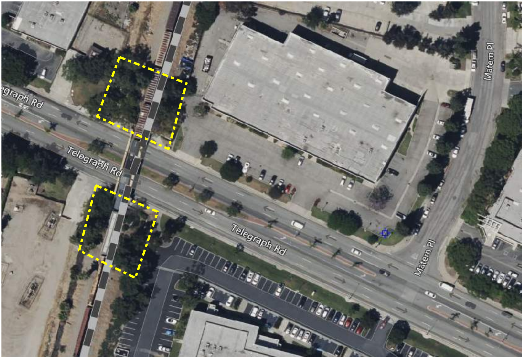
TELEGRAPH ROAD E/O PIONEER BLVD - PLANTER AREAS
